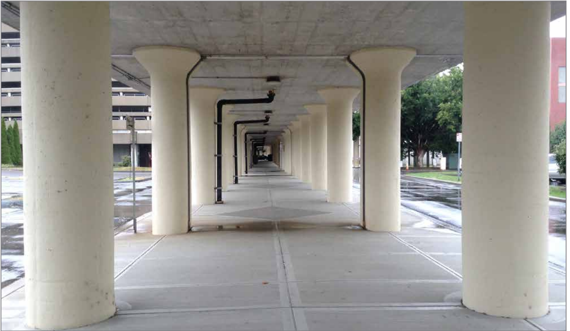
Photo of existing viaduct
