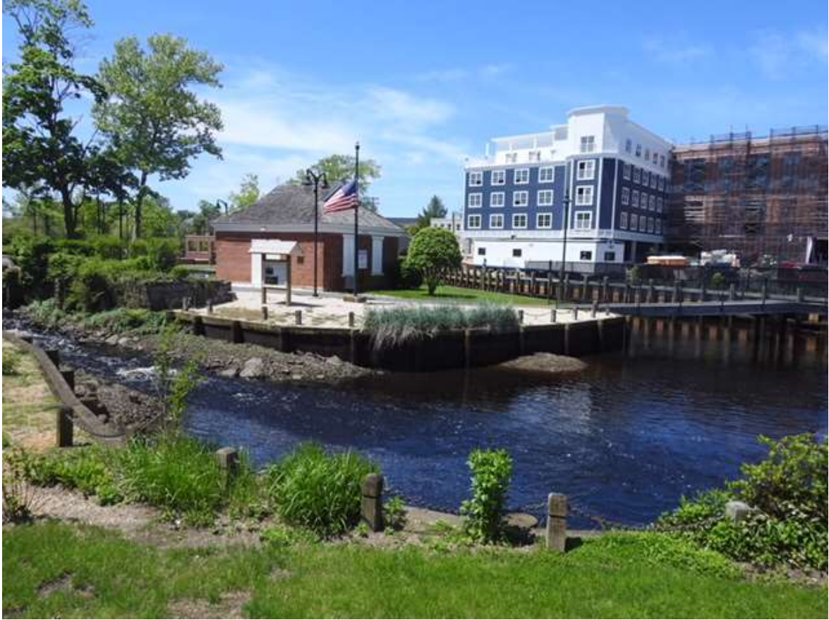
Grangebel Park overlooking new Peconic Crossing, 45-unit affordable apartment with artist residences and gallery
