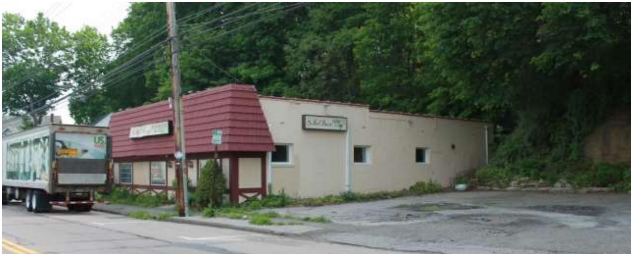
Abandoned Property located in the main Downtown Area. Town has since obtained this property due to delinquent taxes and financed the building demolition in 2016.
