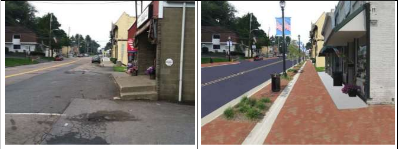
Current condition of street along Elwood Ave juxtaposed with rendering of planned improvements as part of the Elwood Streetscape Project.
