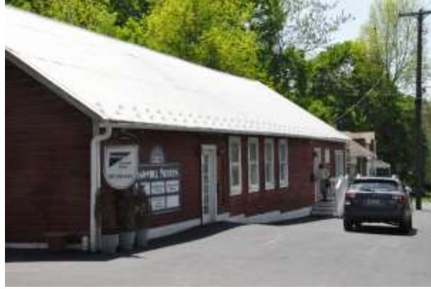
New office complex on Grove Street in former sawmill
