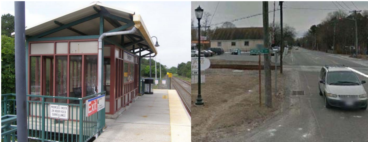
Bellport LIRR Station Waiting Area (left), LIRR Crossing (right)
